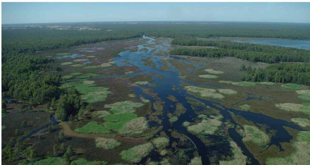
Levees and other structures control water entering the floodplain from Dhungalla. (Photo: Keith Ward)
